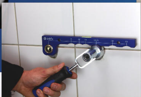
Aligning the S- Connections.
