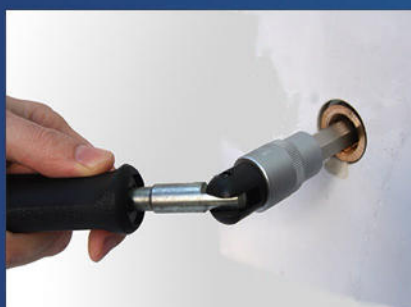
Screwing in and unscrewing Tap extensions.
