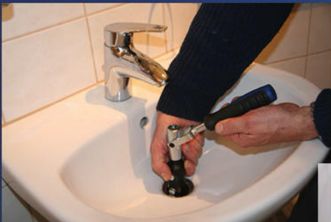
Counterbalance the drain valve.
