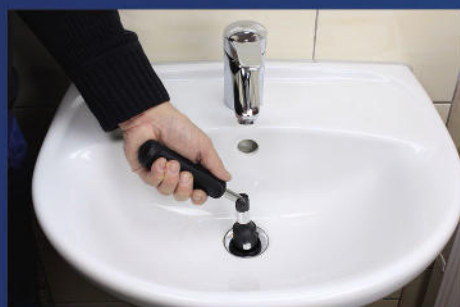
Counterbalance the drain valve.
