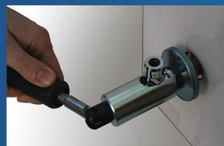
On and unscrew Angle valves.
