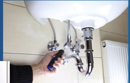
Mount the securing screw of fittings.
