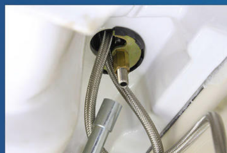
Mount the securing screw of fittings.
